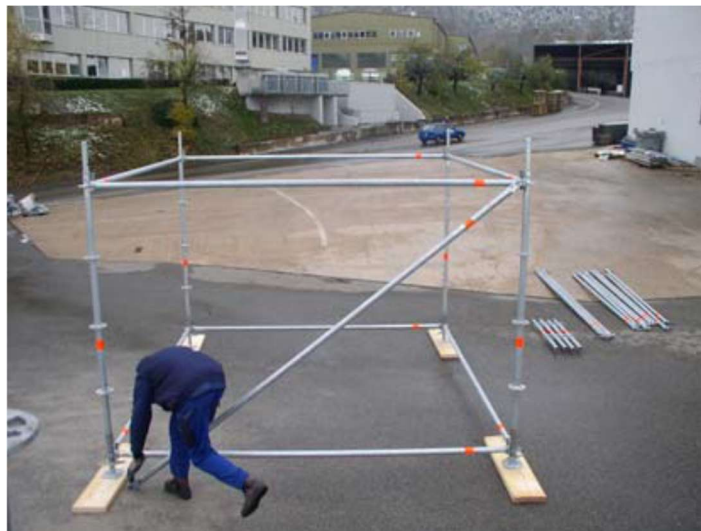
Fig. 4. Assembly of the first horizontal frame
