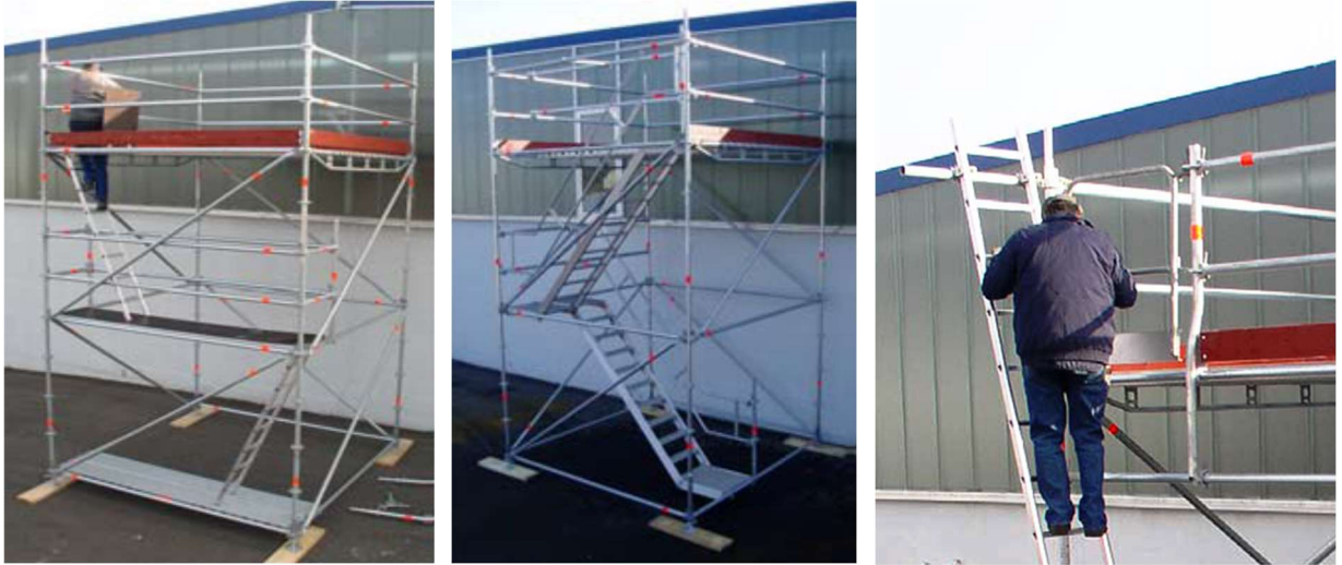
Fig. 5. Examples of installed access means
