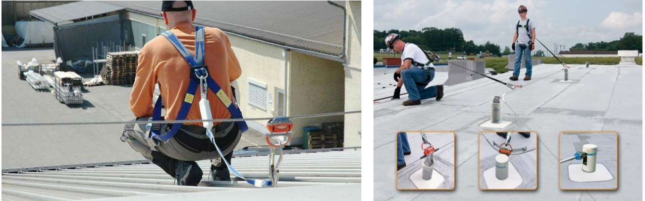
Fig. 2. Examples of horizontal safety systems
